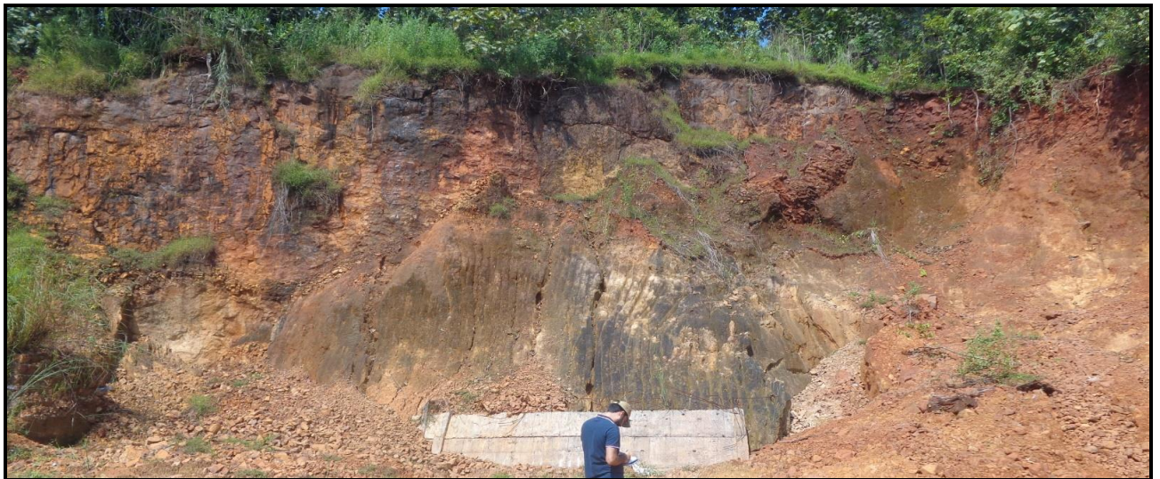
Photo 13: Regolith thickness less than 0.5m along the road connecting Bantval to NH-48
