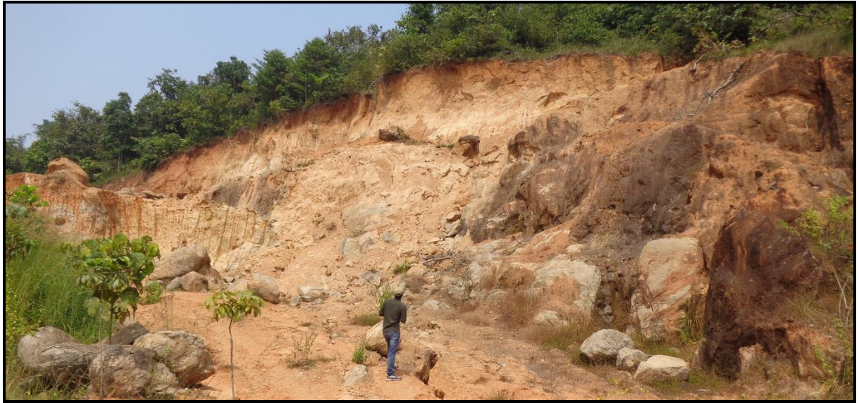
Photo 4: Extensive cut slope along Bantval-Amtadi Road section
