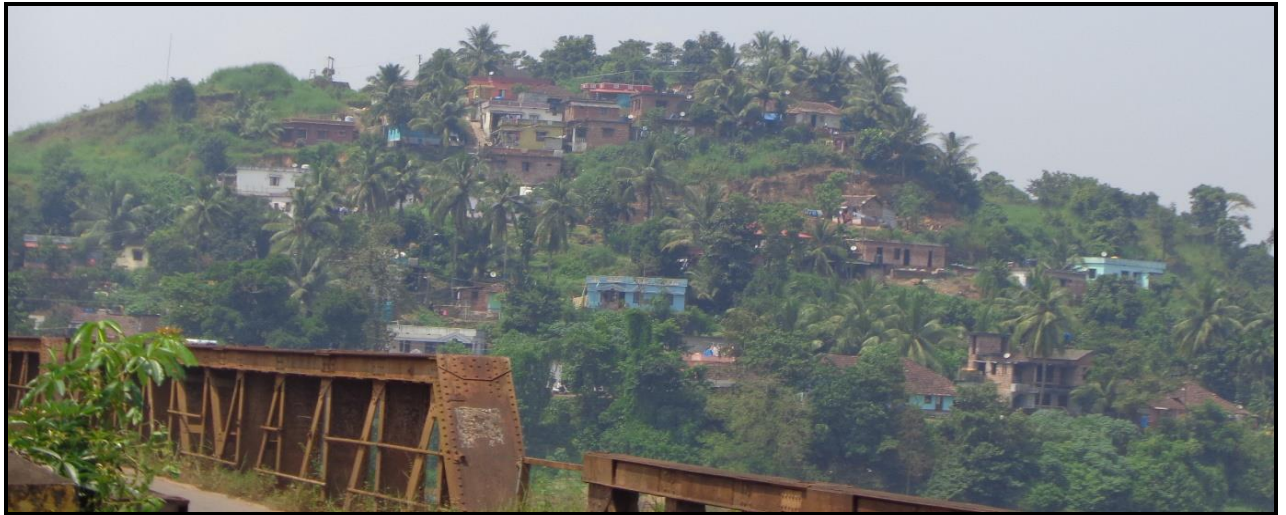
Photo 5: Settlements on modified slope near old road bridge on Netravati river
