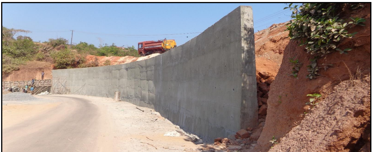
Photo 19: Retention wall being constructed near Vamajoor for prevention of loose material from sliding
