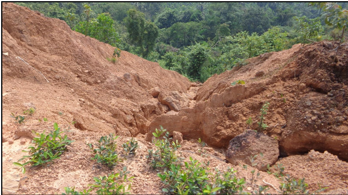
Photo 16: Loose debris dump on the downslope side along the Bantval-Lorettopadavu road section
