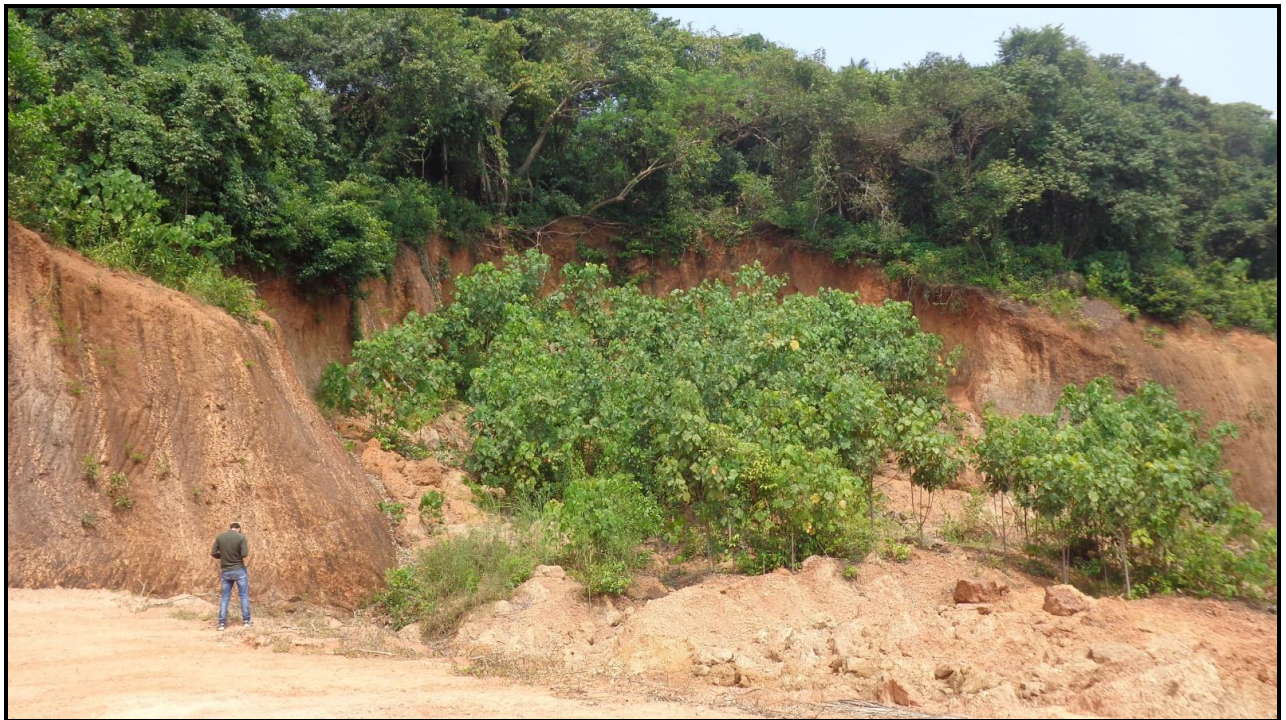
Photo 23: Debris slide caused due to toe removal along Bantval-Lorettopadavu Road section
