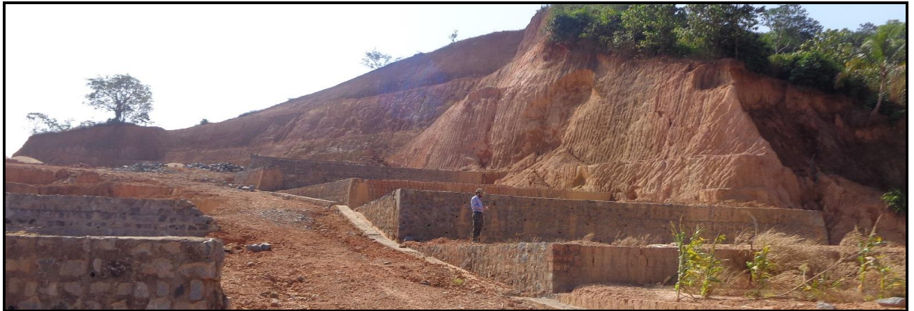
Photo 17: Slope modification for settlement on the road, North of Farangipet
