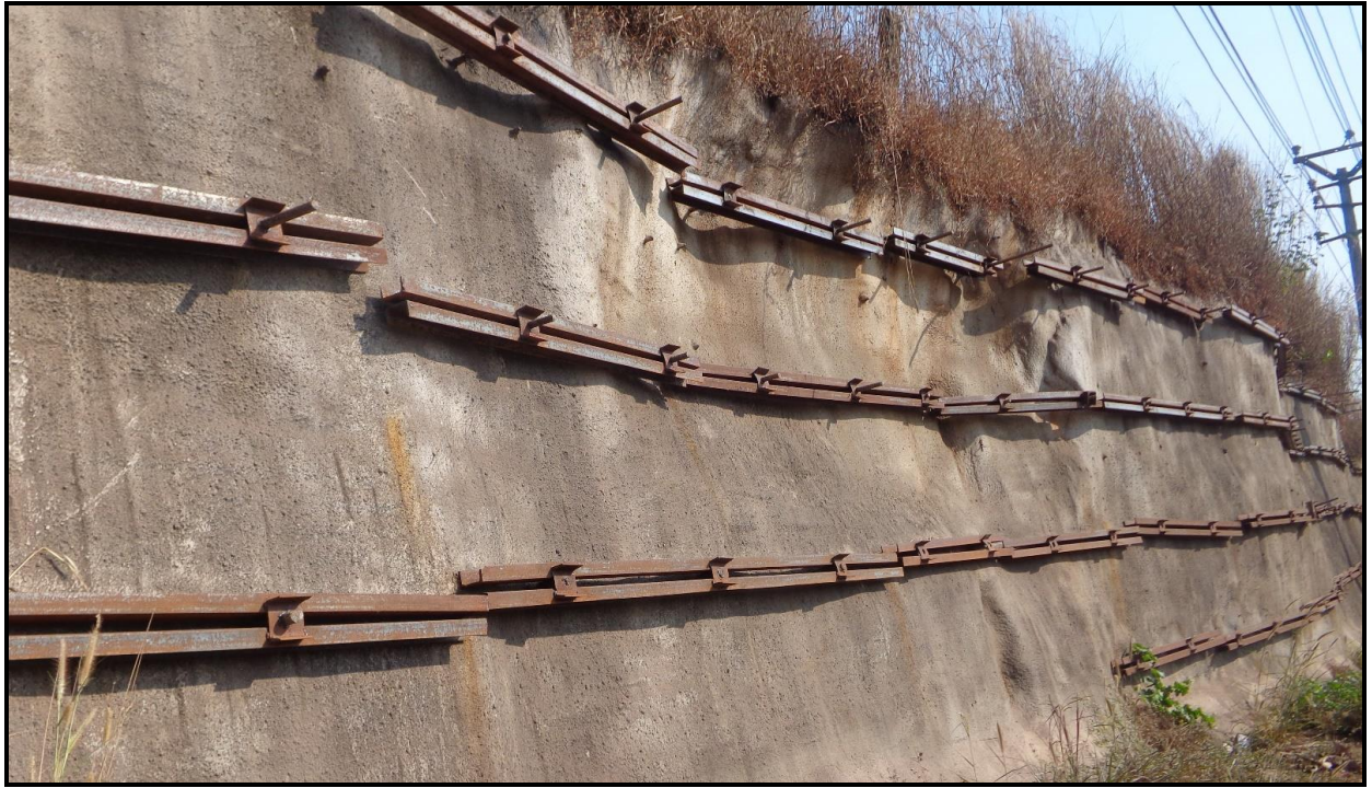
Photo 20: Rock bolting along NH-48 near Padil for stabilizing slope
