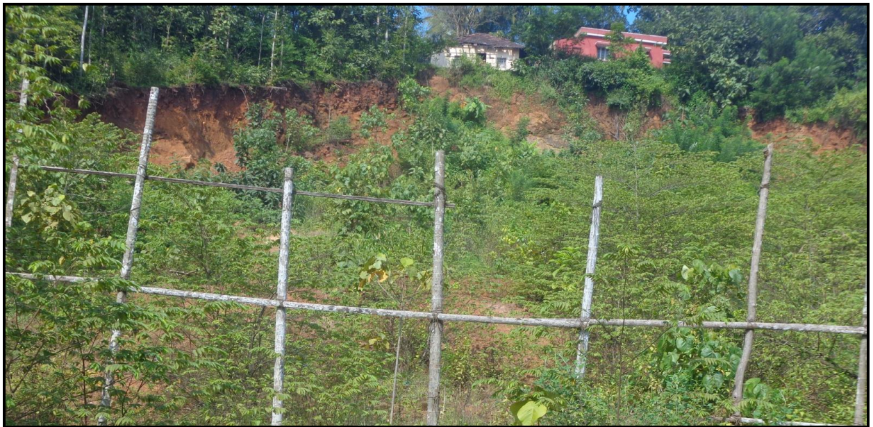
Photo 21: Debris slide initiated by excavation for settlement along the Bantval road connecting to NH-48 (Earlier reported in local newspaper; causes collapse of the houses and loss of life)
