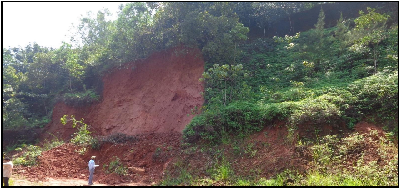
Photo 22: Debris slide initiated by road cutting along the road near Modanthyar
