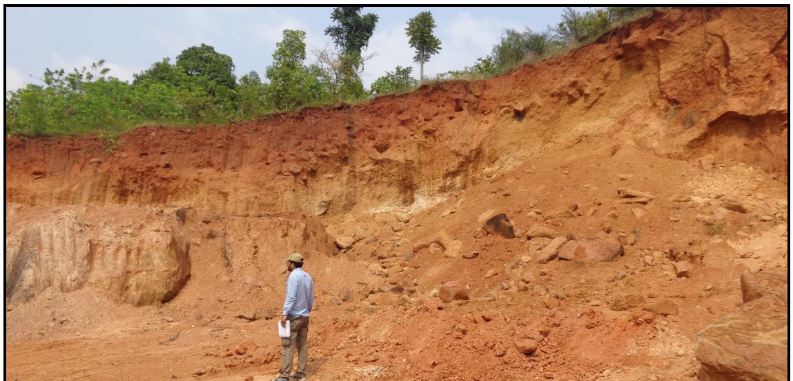
Photo 2: Extensive cut slope in soil along Kalladka-Melkar Road section
