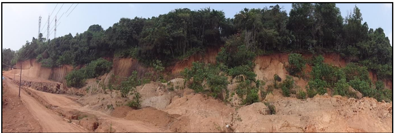
Photo 3: Extensive cut slope along Bantval-Lorettopadavu Road section
